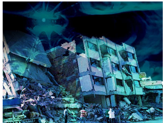
Fig. 10. Homes crumbled under the intense Kashmir Earthquake
